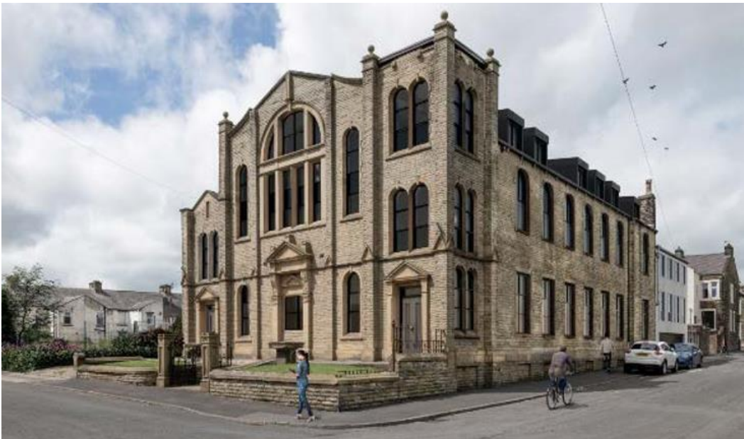
Visual showing the proposed alterations to the elevations fronting Claremont and Tabor Streets
